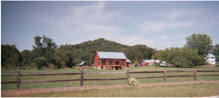
This barn remodel, now used for residential use, illustrates one way to preserve rural heritage by maintaining traditional structures and design elements.
